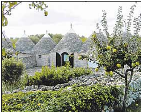
Legend has it these mortar-free stone dwellings, called trulli, were designed to be quickly dismantled when tax authorities were in the area. When they left, locals rebuilt the houses.
